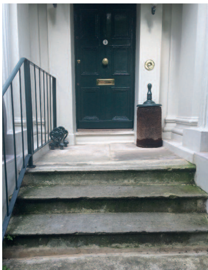
Original Portland stone steps on Ladbroke Terrace.
