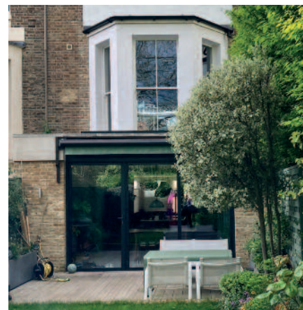
The same house after the lower part of the newly rebuilt bay was removed and replaced with a glazed extension.
