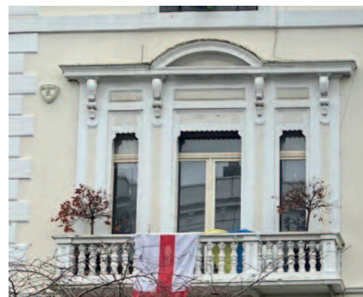
Former balcony and windows with awning covers on 41 Chepstow Villas
