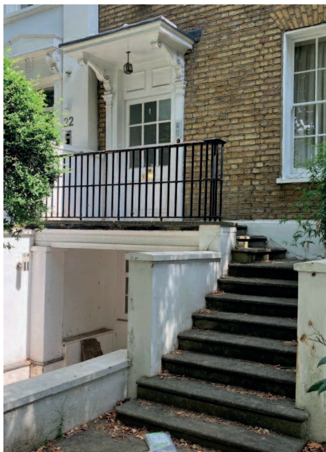
22 Ladbroke Grove where the steps were moved and a new main entrance was built under the original front door.
