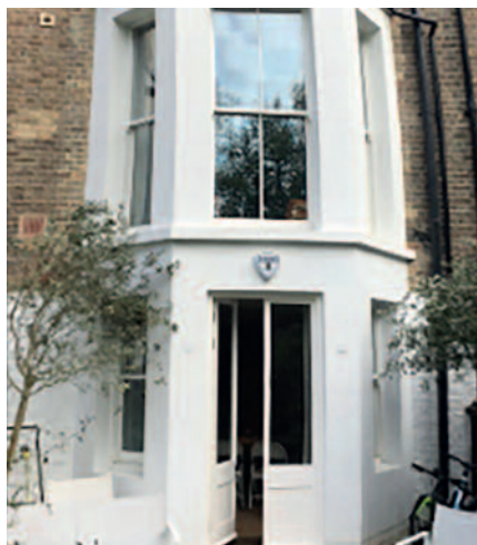
The same house after the bay was restored in 2016.
