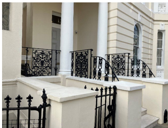
Decorative ironwork on porches in Stanley Crescent
