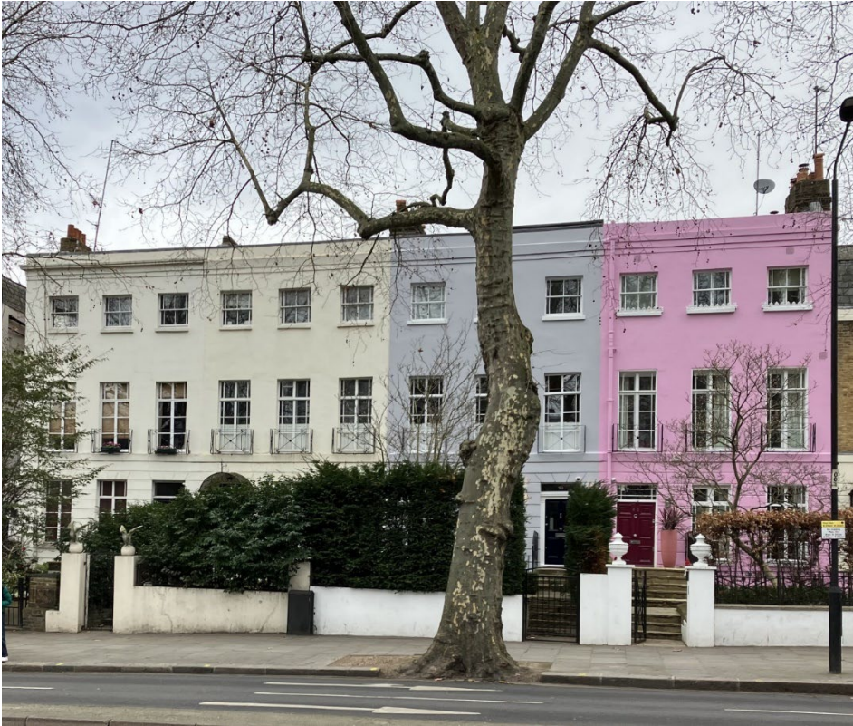
These (on Holland Park Avenue) are some of the earliest houses on the estate and are full stucco
