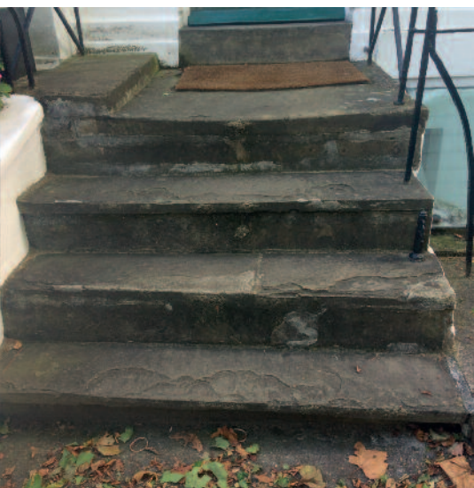
Well-worn probably original steps at an 1830s house in Ladbroke Grove. These early steps were square cut; later bevelled or bullnosed edges were used.
