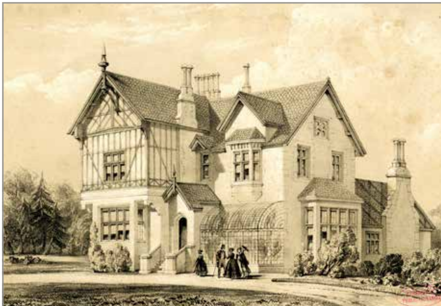
Former "Swiss Villa" in Kensington Park Road
