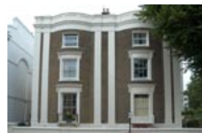
12-14 Clarendon Road - a building that relies on the contrast between brick and mortar stucco for its charm. Copyright Thomas Erskine
