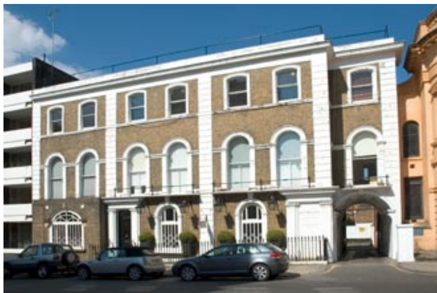
92-96 Kensington Park Road. Photo © Thomas Erskine.
