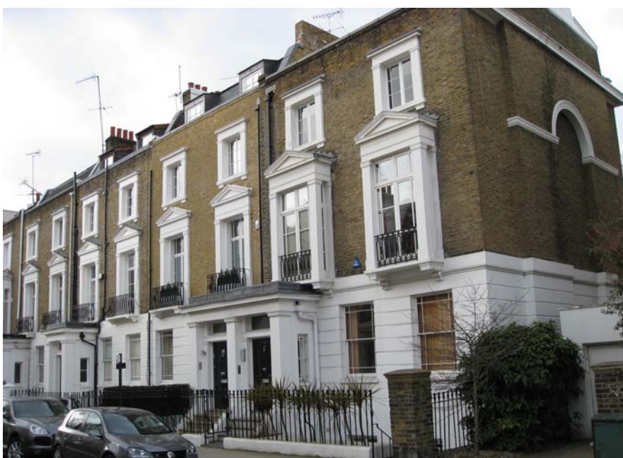
Below the same terrace in 2009 after removal of the paintwork on No. 37
