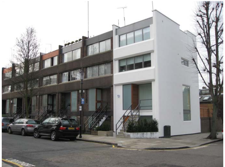
No. 11 Clarendon Road, the end house of a terrace built in the 1960s and recently stuccoed over. The terrace is just outside the Ladbroke conservation area.
