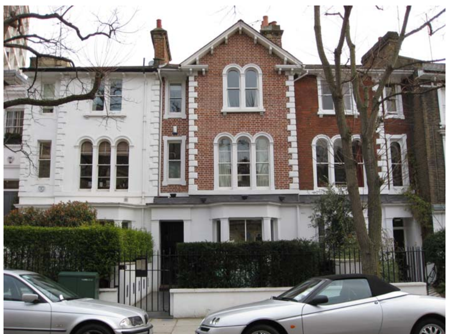
21, 23 and 25 Ladbroke Road, a symmetrical trio with unusual red-brick upper floors, marred by the addition of stucco to No. 21. ©Thomas Erskine
