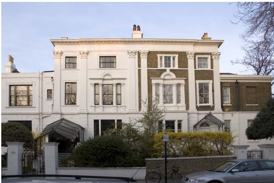
16 and 18 Lansdowne Road, with the brick-work on the left-hand house fully covered in stucco. (Photograph ©Thomas Erskine, 2006.)
